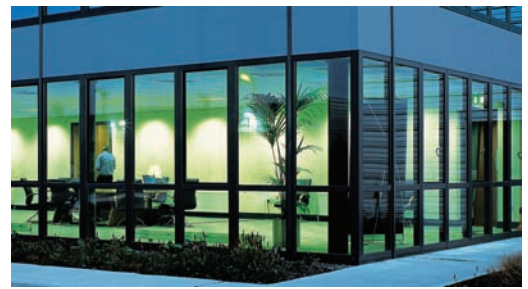
New technology: glazing bonded into the sash improves static and saves material.
