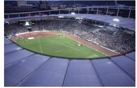
For maximum stress with little material: the roof of the Gottlieb-Daimler Stadium in Stuttgart/Germany.
