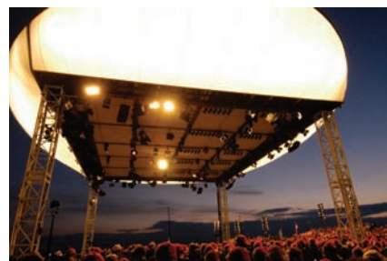
Exceptional: PVC-coated membrane canopy for Pope Benedict during the World Youth Day 2005 in Germany.
