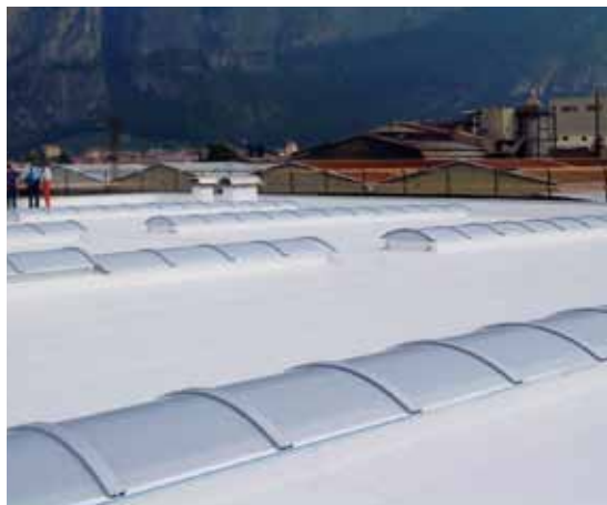
Industrial Building (Italy): RENOLIT ALKORBRIGHT
