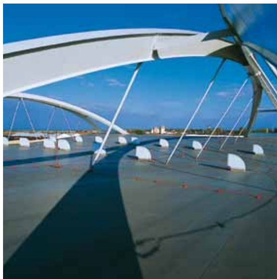
Transport station (Czech Republic)
